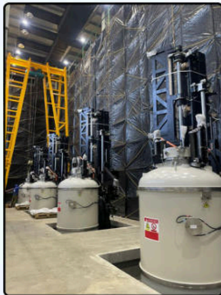
Ingot Pullers Installation
