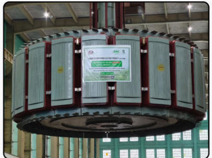
Rotor Lowering at Unit 5
