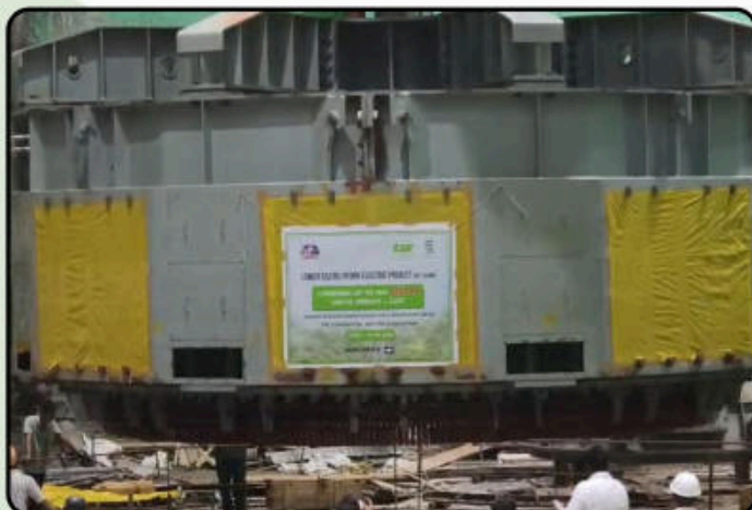
Stator Lowering at Unit 6
